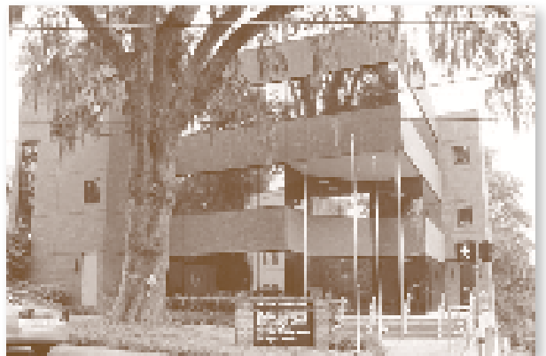
FES Headquarters, a three-story, 19,300 square-foot building with two levels of parking was completed in 1992. In August 2007, the building was dedicated to John A. Grant Jr. PE.
